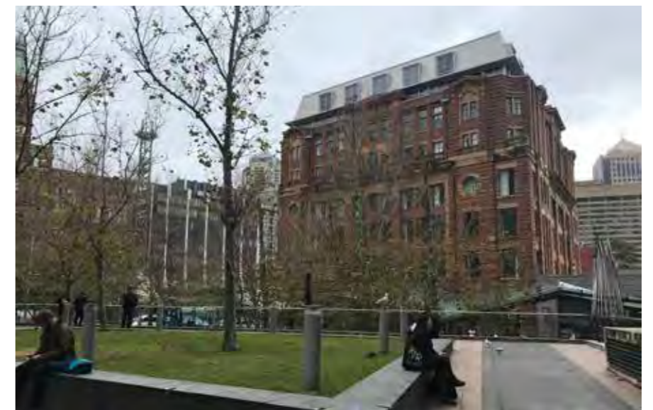
View towards the southern facade of the heritage former Parcels Post Office Building.
