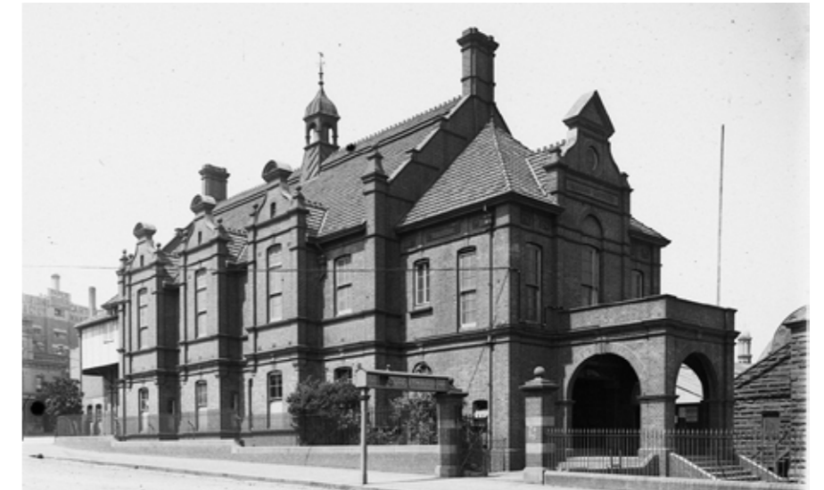
Railway Institute Building 1919 (Source: NSW State Archives)
