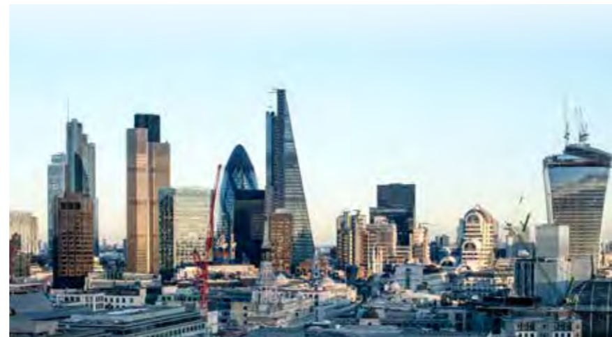
Potential higher density development, establishing a visual marker for Central Precinct and contributing to the future skyline of Central Sydney.
