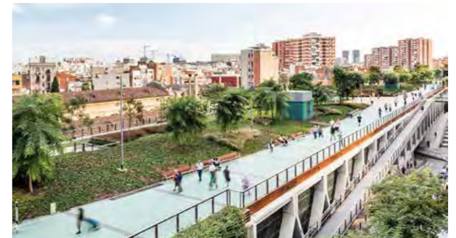
Provide green connections over track, linking Surry Hills and Prince Alfred Park to Chippendale and Ultimo across Sydney Yards.
